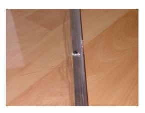
Adjacent angles are fixed by a bolt at the corner of the cover. This picture also shows the gap between the edge of the plate and the vertical side of the end angle.
