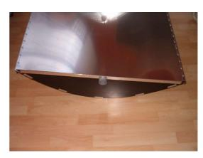
Use a flexible adhesive ribbon to close the gap between two adjacent joints. Here the adhesive ribbon is of the same color as the plates, so it is not easily distinguishable.
